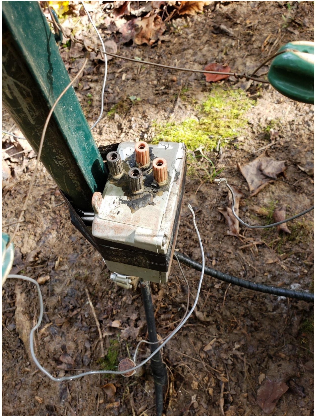
Figure 3. N4GGG's K9AY Loop outdoor termination box with antenna wires disconnected.
