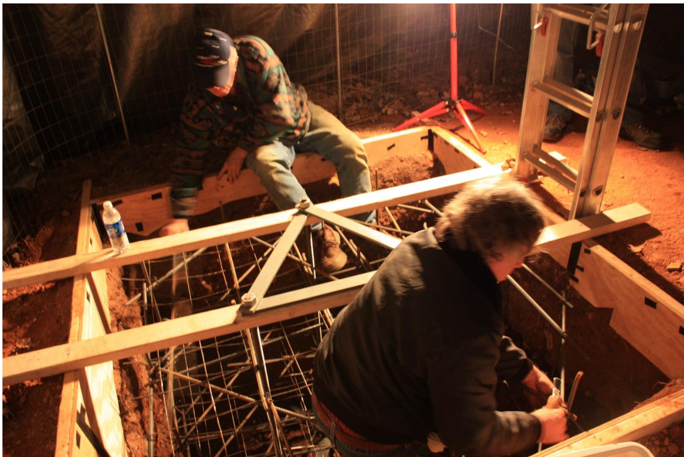
Installing rebar on a cold night: Gene - W5LE (SK), Gary - WB4SQ
