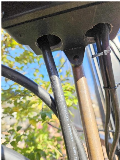
Figure 3 The bottom of a NEMA box in use outdoors at N4GG. The bottom of the box is wide open.
